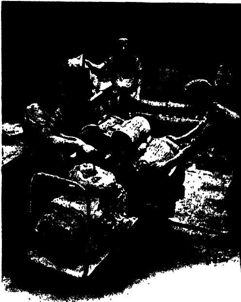
MILLING AND PUGGING CLAY, BRITANNIA POTTERY, GLASGOW.
